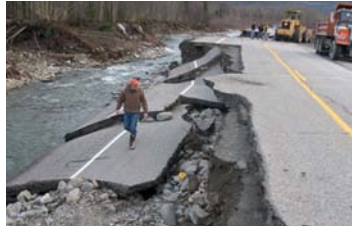
Melting ice in permafrost areas such as Alaska is catastrophically collapsing paved roads and buildings.
