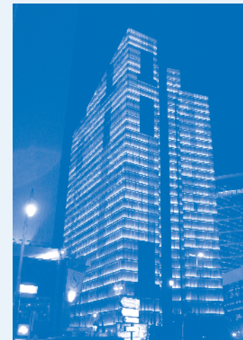
LED media façade of the Dexia (now Rogier) Tower in Brussels (2006).
