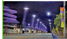
2000 Olympic Boulevard Light Towers, Sydney
