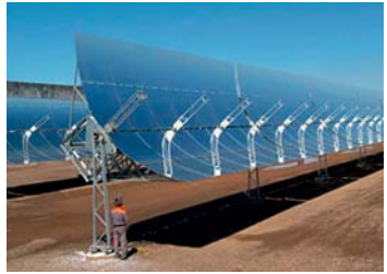
Large arrays of solar thermal collectors are humanity's best future source of renewable power.
