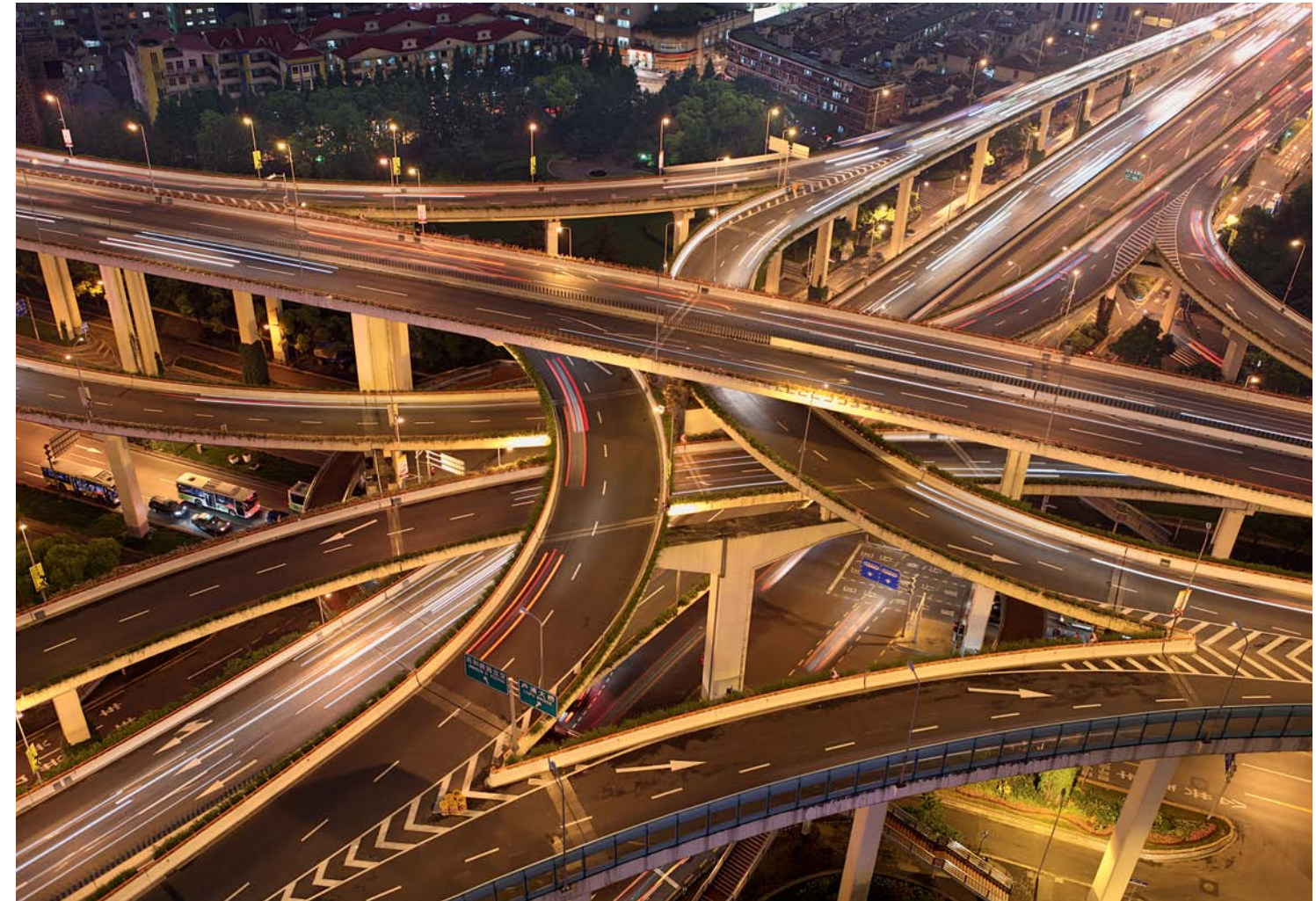
Infrastructure of the fossil fuels era: motorway spaghetti in Shanghai (photo SevArt/PicFair).
